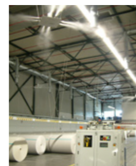
Roll-carrier level with TurboFog 32 high-pressure humidification
